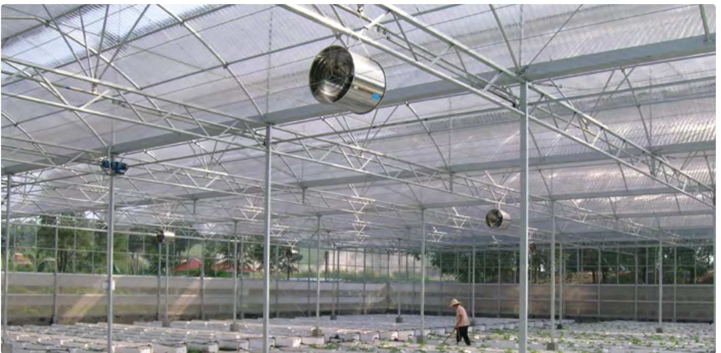
Arched Roof - China
