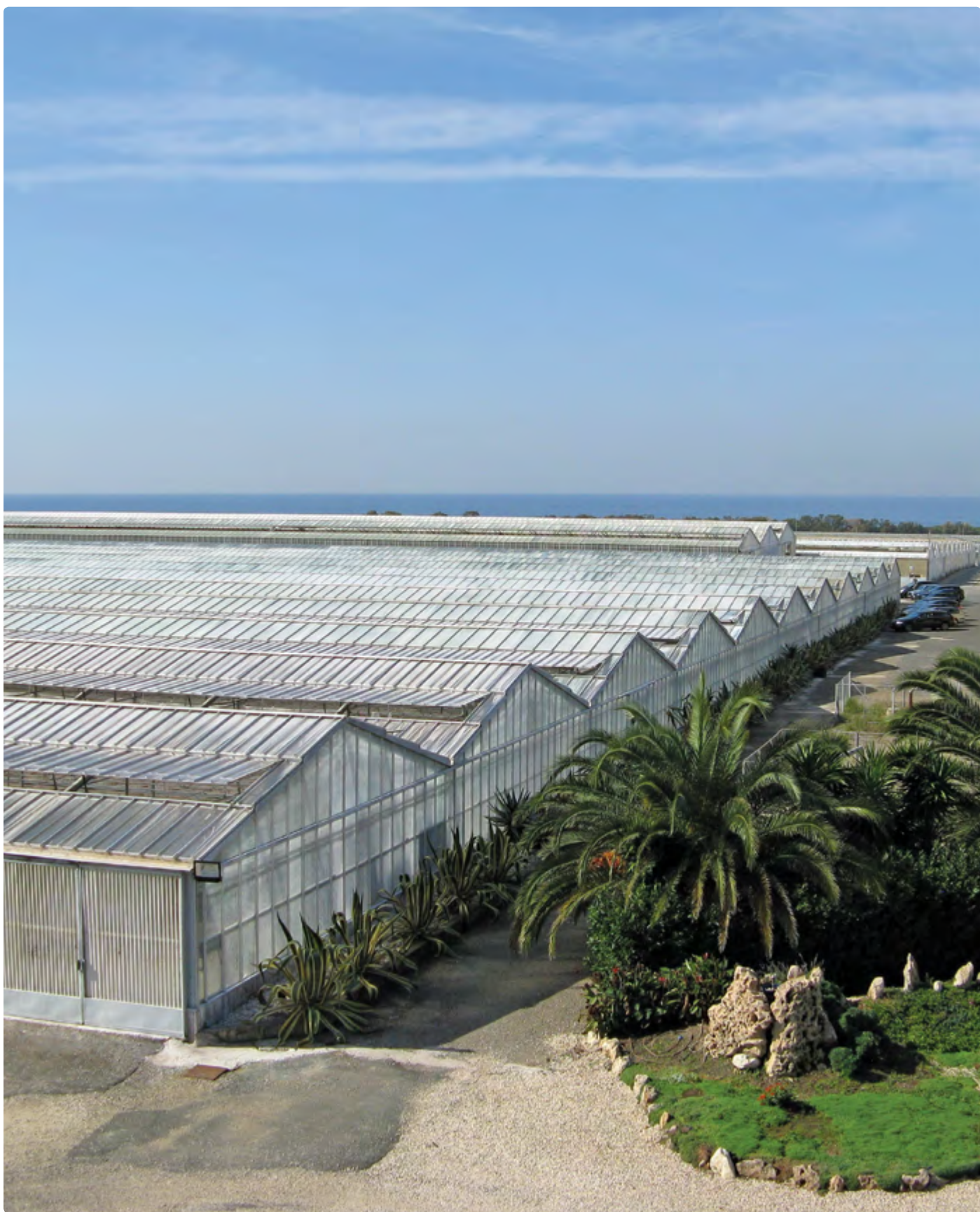
Custom Made SUNTUF Plus for Glass Replacement Project - Southern Italy
