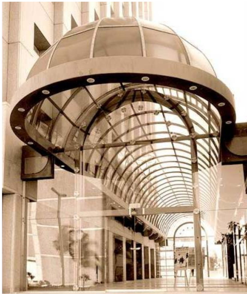
Figure 10. Typical Curved PALSUN Glazing, Skylight Canopy over Main Entrance to Office Building & Shopping Arcade. Cold-Curved, 6mm Clear PALSUN. PALGARD Should not be Used as Curving would Damage the Silica Coat.
