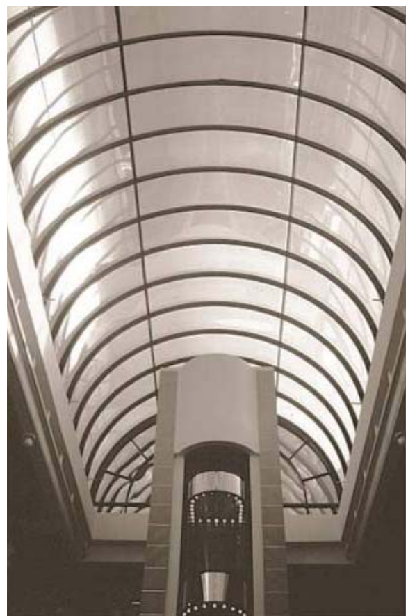
Figure 29. Heavy-Duty PALSUN Glazing & Specialized Aluminum System with External Condensation Channeling on a Vaulted Skylight over a Shopping Mall.
