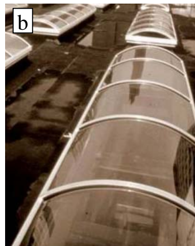
Figure 30 a,b. Cold Curved PALSUN Glazing a. Cold Curving Process (Top) b. Cold Curved Glazing in Skylights (Bottom)
