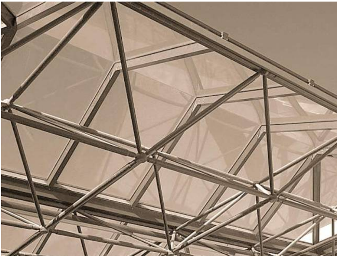
Figure 9. Typical Flat PALSUN Glazing, Skylight Canopy over Main Entrance. ORT Technical College, Natanya, Israel. Cold-Bent, Angled Frameless Ridge, 6mm Clear PALSUN. PALGARD may be Used, but Bending at the Ridge will Damage Silica Coat along Bent Line.
