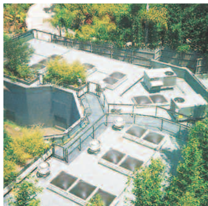
A typical skylight application at The San Diego Zoo.
