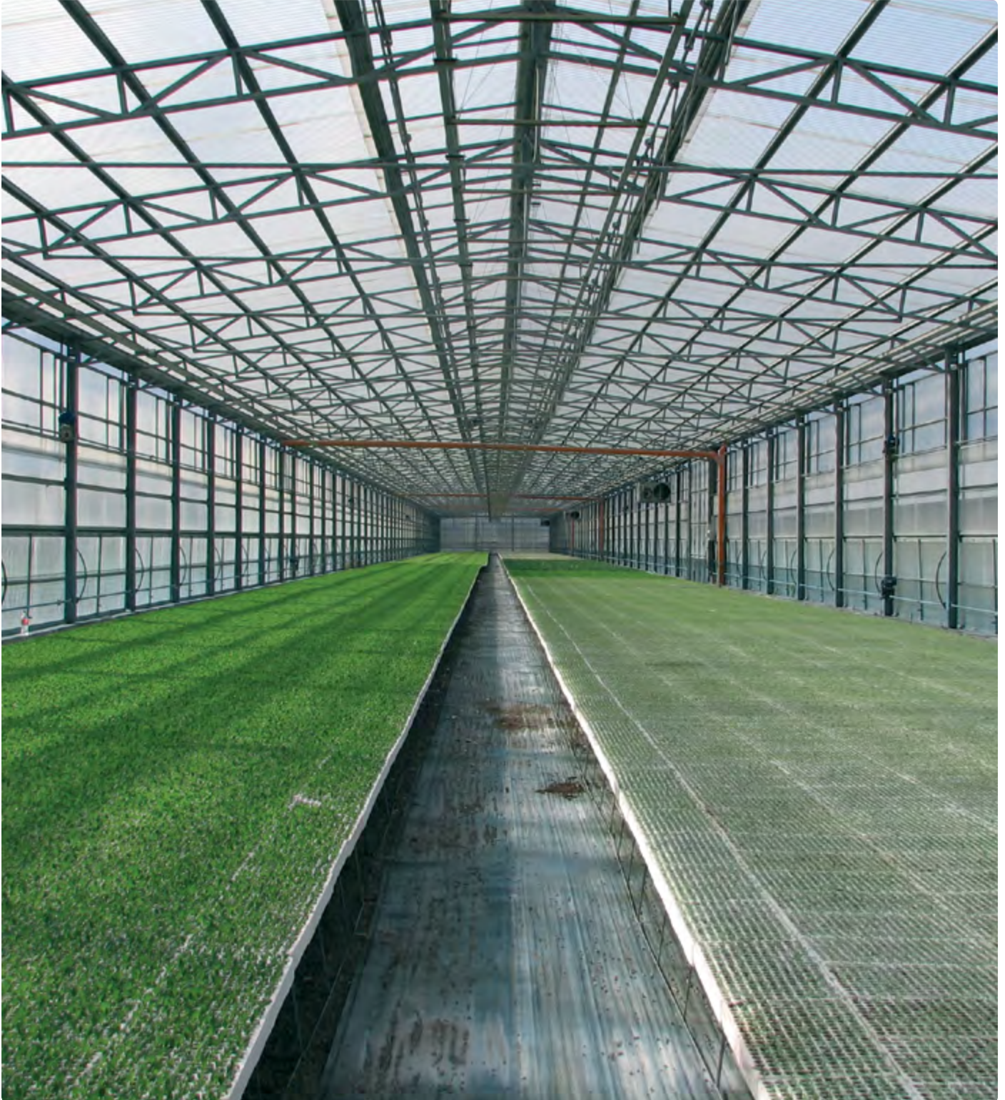
Double sloped roof and walls - Southern Italy
