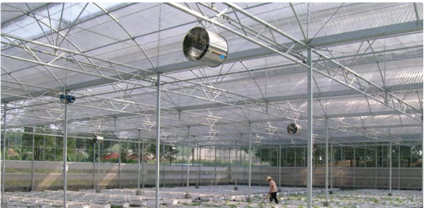
Arched Roof - China
